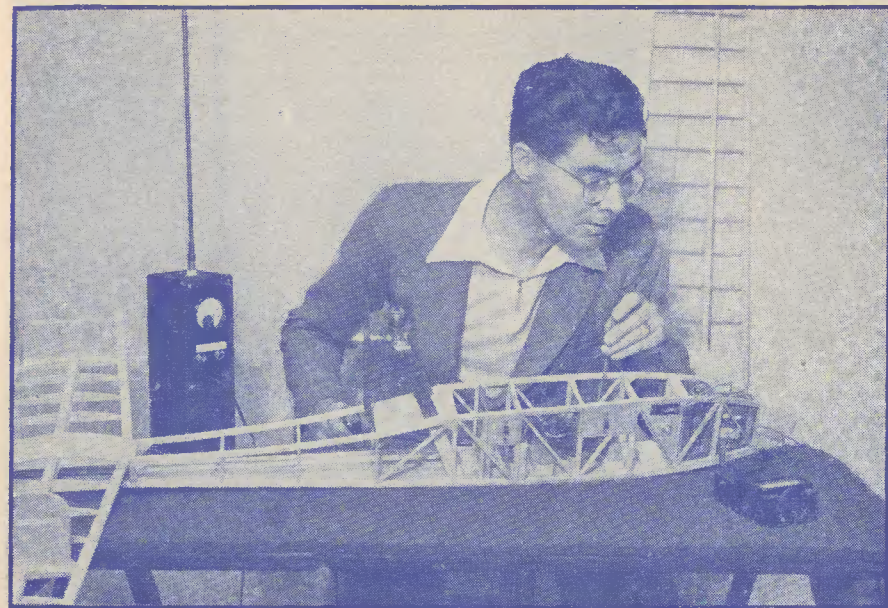
Fig. 9. This illustration shows the receiver being tuned, and gives an idea of the size of the model. In this case a large meter is being used, but on the flying-field a smaller type is employed, as shown in Fig. 11.
